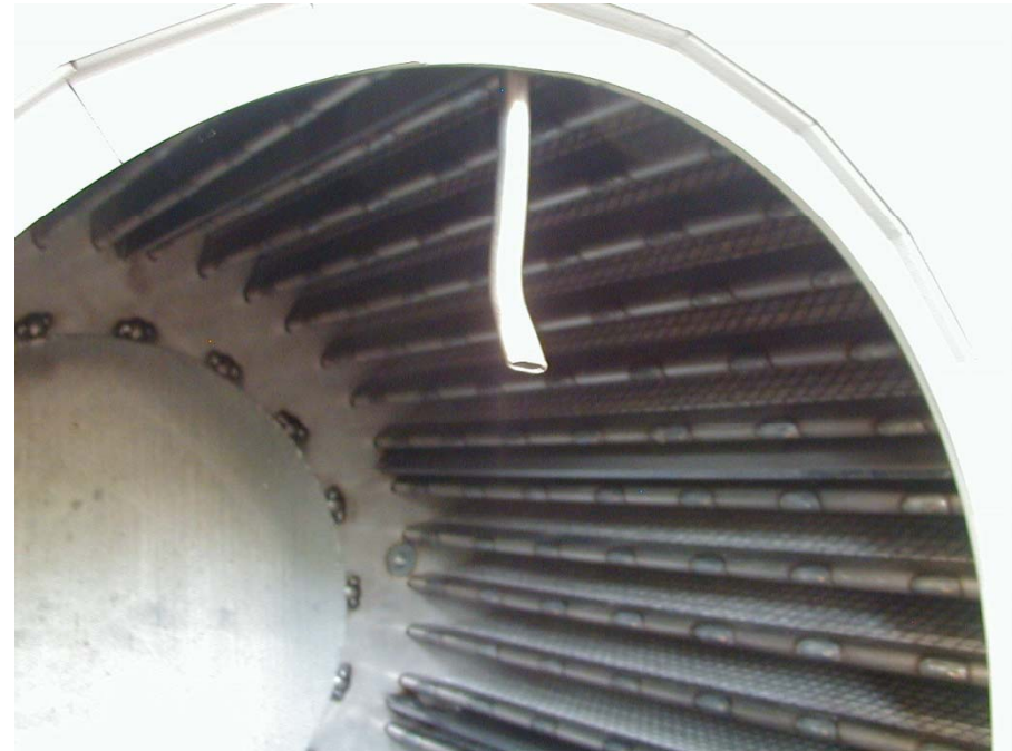
Inner section of silencer with washing nozzle
