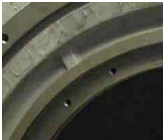
Recess in the outlet casing
